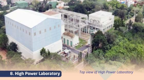
**Test Facilities:** Short circuit testing of Power Transformers, Instrument Transformers, Switchgear & Control gear and other allied power system equipment. Lab is equipped with mechanical & switching performance test facilities for switchgear equipment.
