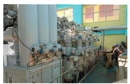
A view of the test undertaken on the 3 phase 245 kV, 2000A, GIS Breaker
